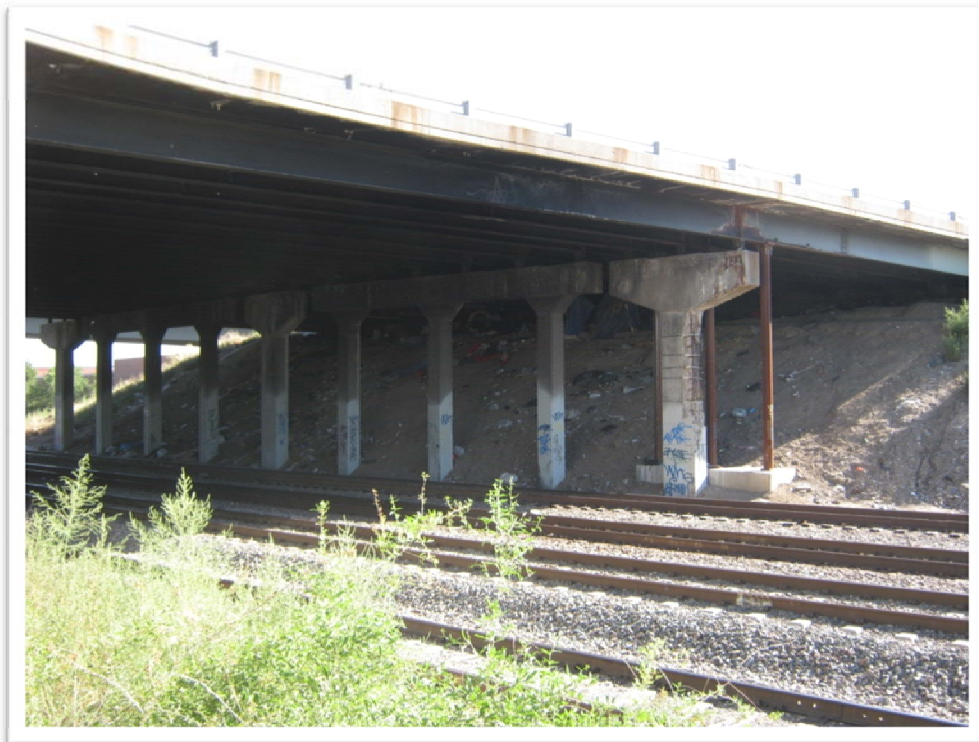
Photograph 2 – Elevation of existing pier looking east
