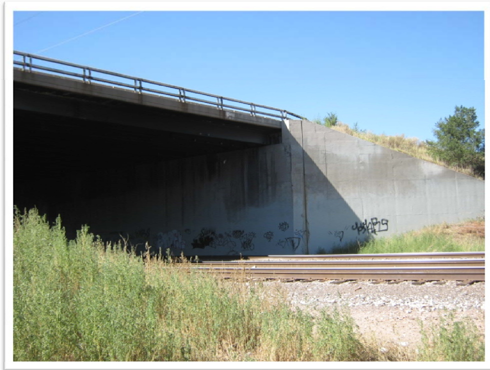
Photograph 3 – Existing abutment looking west
