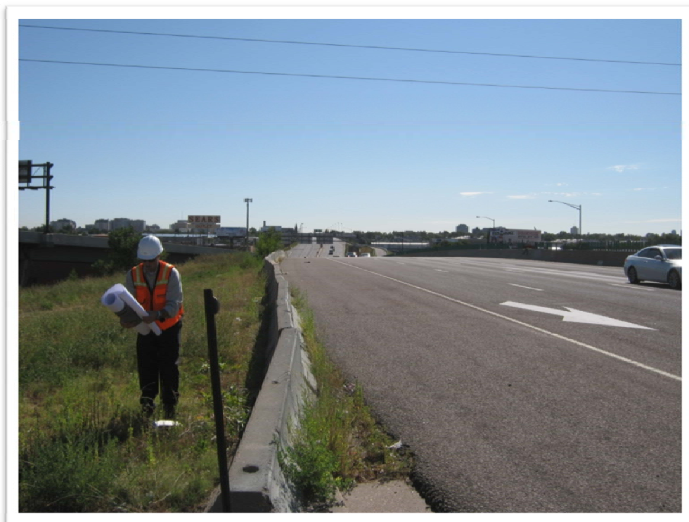
Photograph 4 – West approach looking east
