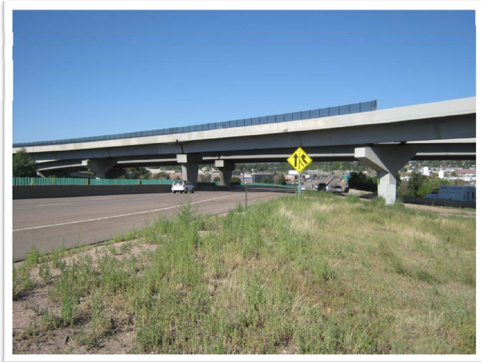
Photograph 6 – Existing US-6 under Structure F-16-OL looking west
