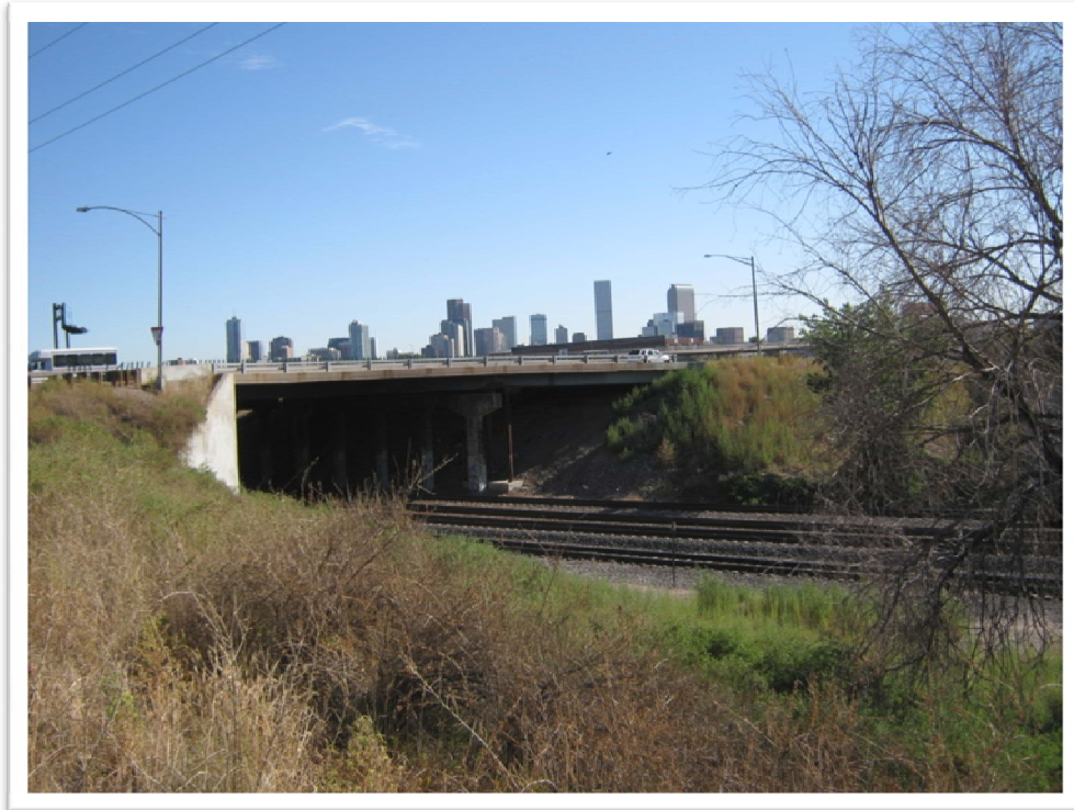
Photograph 1 – Elevation of existing bridge looking north
